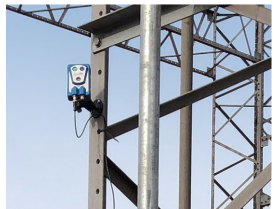
Figure 1 – IM500 thermal plus visual sensor module can be installed close to high power.
